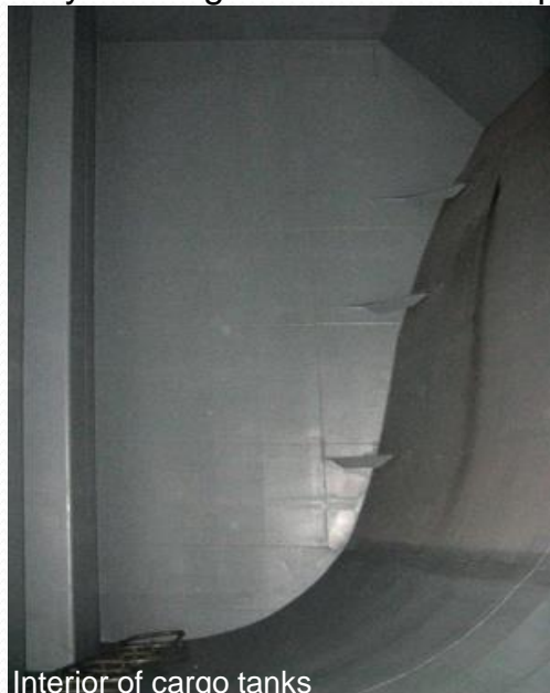
Interior of cargo tanks
